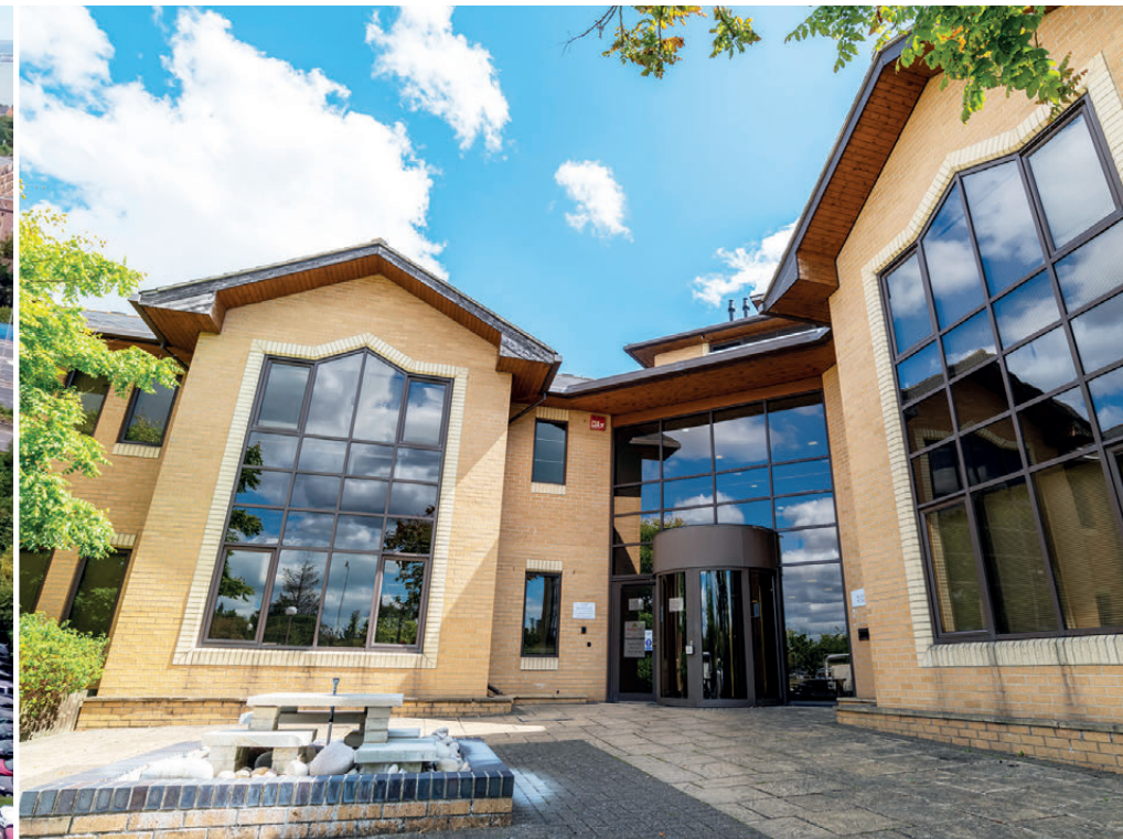
Entrance to the main reception of Harbour Court.
