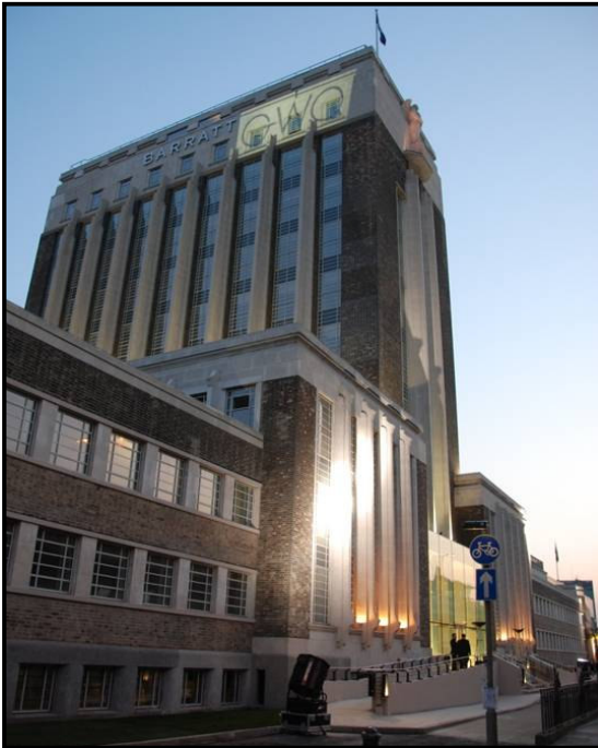
Photograph of Wallis House of which subject space forms part
